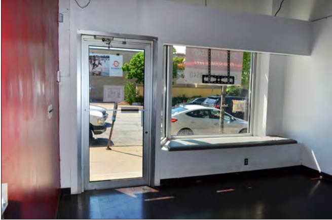
storefront window on Hennepin Avenue
